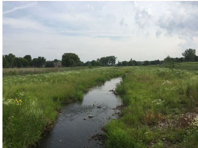
Woods Creek Reach 3 restoration in Algonquin
